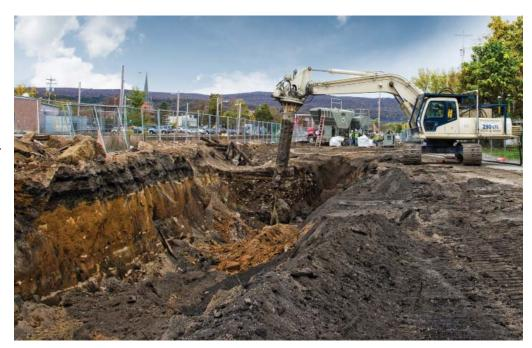
Utilizing a method called deep soil mixing, crews prepared 50 ton batches of bentonite and cement in an on-site concrete silo and then injected the mix into the ground simultaneously with a soil drilling process. As a result, the concrete mix immediately filled the void created by the drilling operation.
