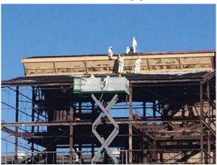
eighty feet in the bitter air and against deep blue skies, asbestos workers carefully remove panels of ACM, lower them to
