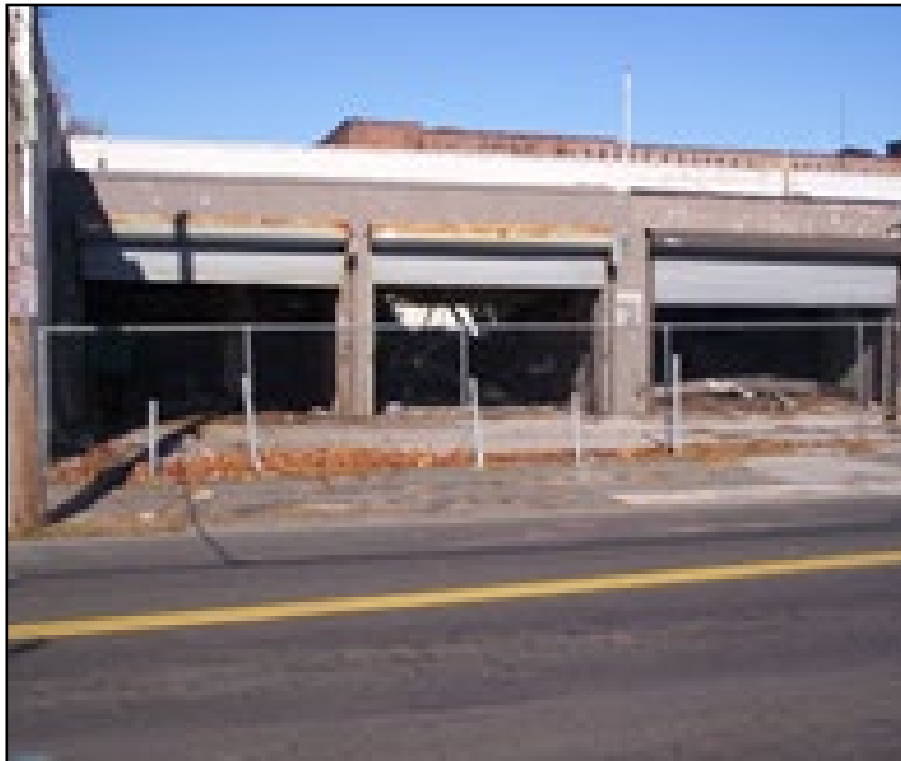
A collapsed roof containing ACM and a common wall complicate demolition efforts. Upper right: completed project.
