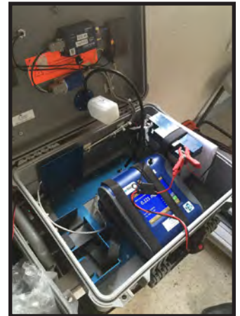
A remote monitor captures real-time data on weather and gaseous fumes.
