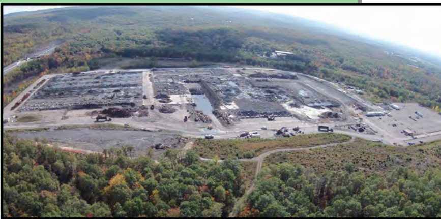
Only stockpiles remain where former factory stood.
