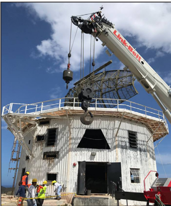
Crews prepare to remove radar antenna.
