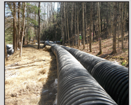
SCE pipelines temporarily divert an impacted stream.
