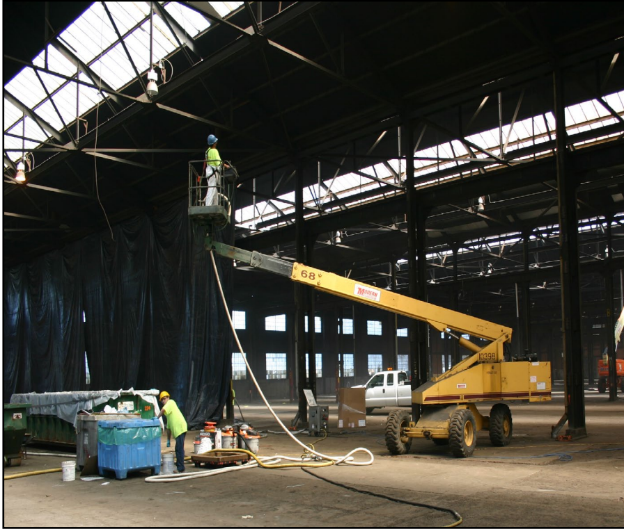
The interior of one of nine bays - each 440' long.
