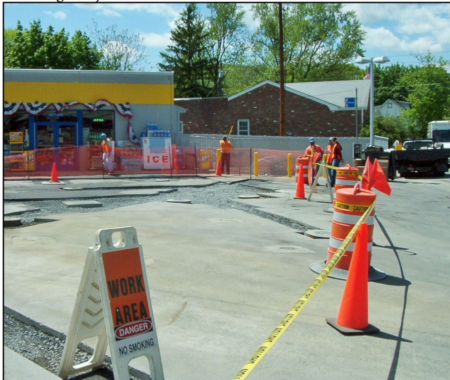
A portion of the 450' trench network.
