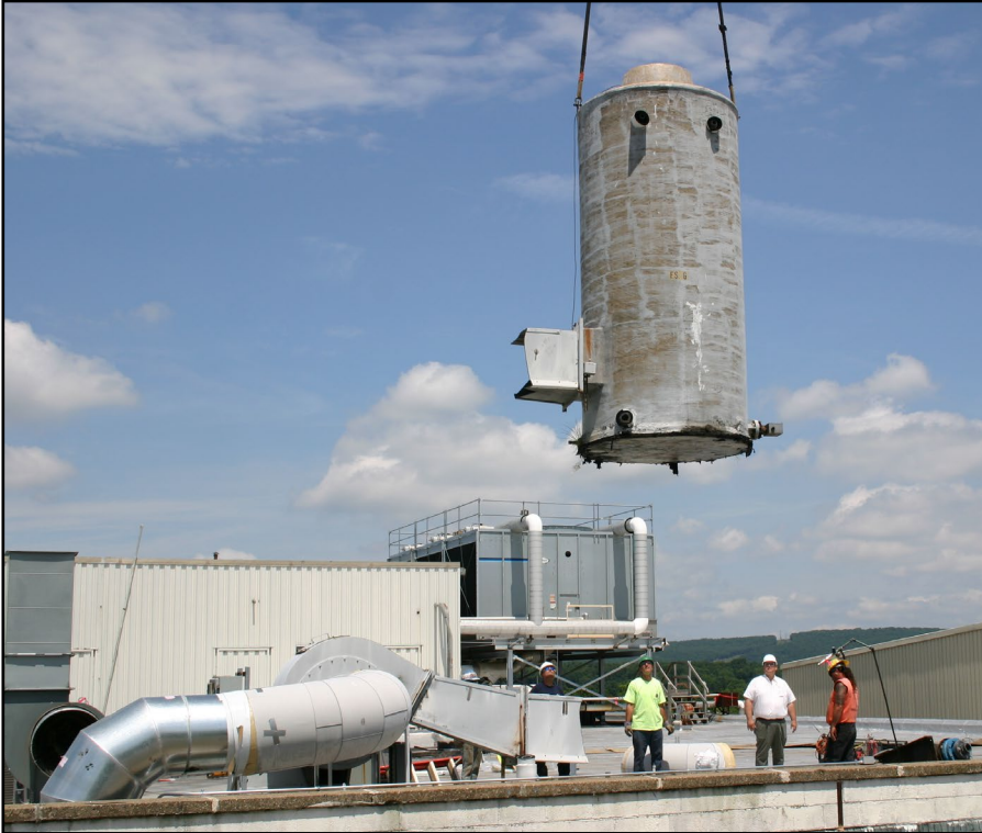
A crane removes a portion of the penthouse air handling system.
