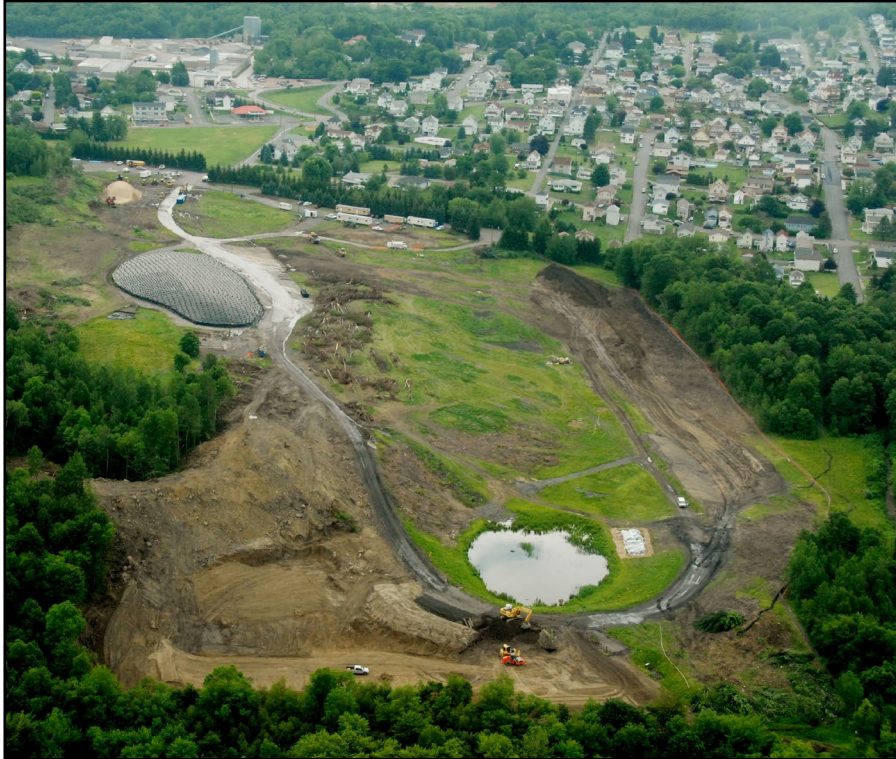
Aerial View: Former battery recycling facility.
