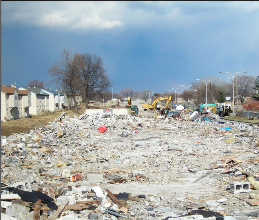
Demolition clears the way for a new development.
