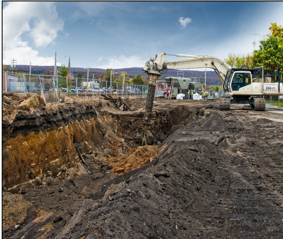
Deep soil mixing equipment mixes soil and concrete to form a barrier slurry wall.
