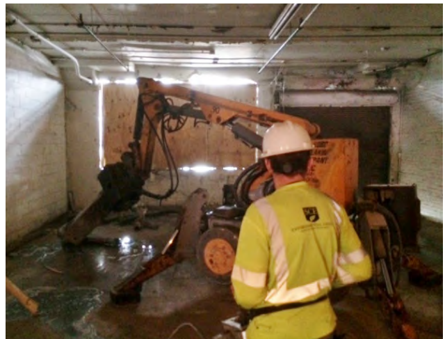
Operating a remote controlled demolition robot equipped with hydraulic shears, an SCE crew member stays out of harm's way as pipes are cut from the ceiling.
