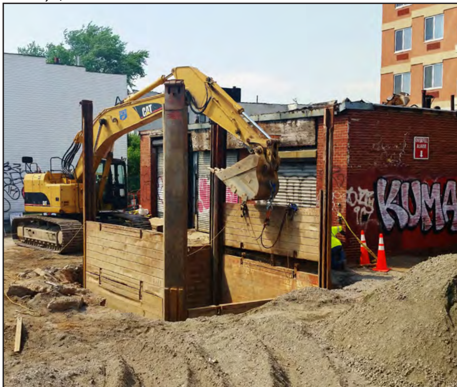
An excavator installs a slide rail as part of a 35' deep excavation.
