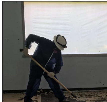
Buildings to be cleared for the new gym.
